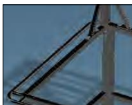
Standard handrail all around the attachment
