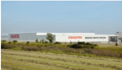
Spare parts centre
