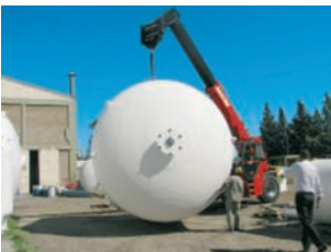
MHT: unloading of a tank on a base
